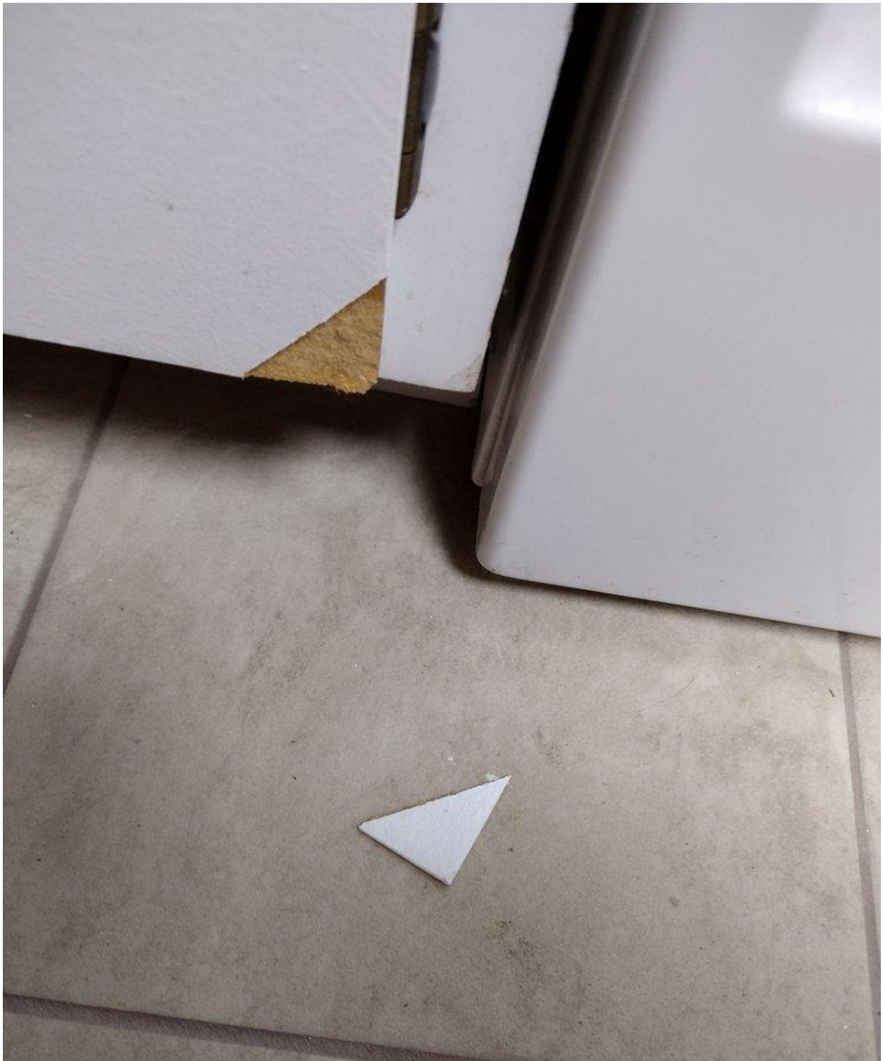
Broken kitchen cabinet, Photo 1.
